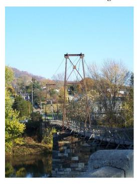
Main Street - Buchanan Swinging Bridge – The Buchanan Swinging Bridge is the most recognized architectural structure in Buchanan. The Bridge is 366 feet long, 57.5 feet tall and the only one of its type to cross the James River. Portions of the bridge date back to 1834 and have witnesses Hunter's Civil War Raid, the rerouting of U.S. Route 11, and numerous floods.
